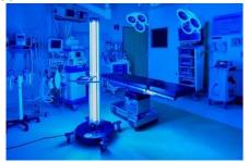
UV-C disinfection using ultraviolet (UV-C) shortwave light incapacitates microorganisms by destroying their DNA.
